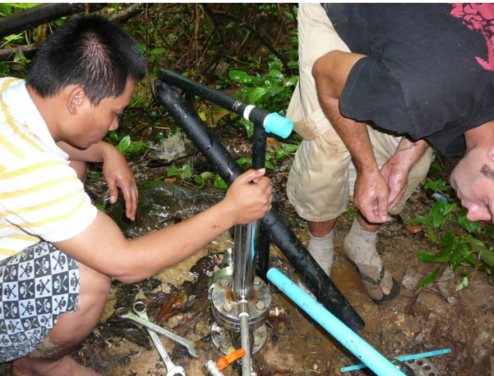
Mounting the pump
