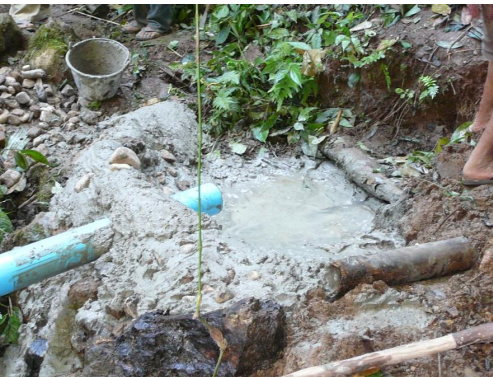
Building the dam
