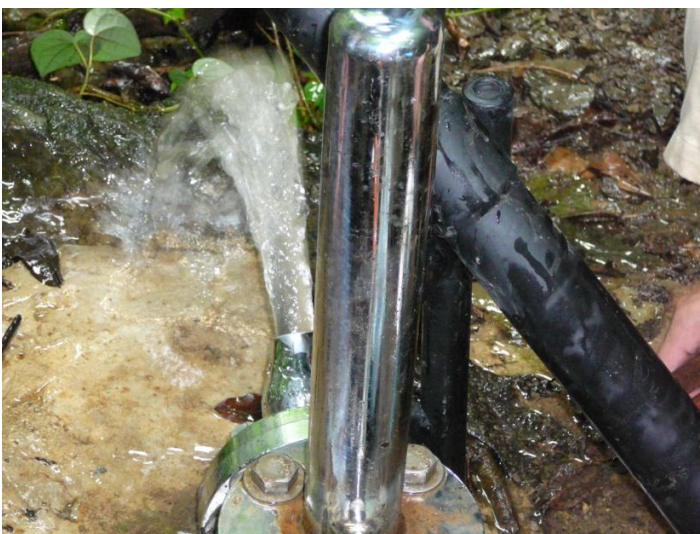
Checking the proper operation of pump and automatic starter device
