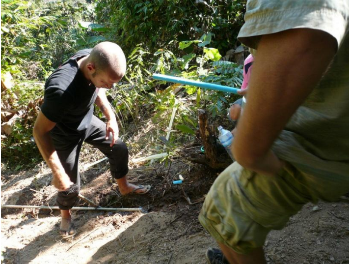
Installing the delivery pipes
