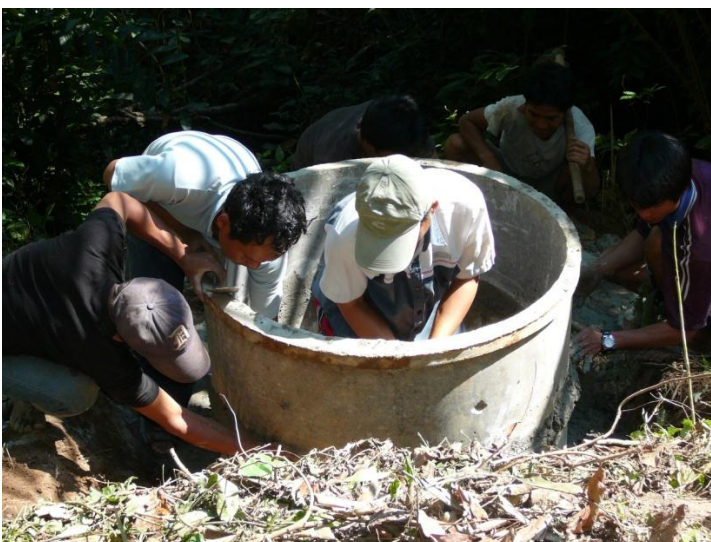
Building the collection tank
